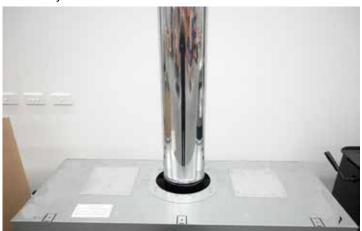
4. Insert the 9" & 11" galvanized flue skin fitted with aircooling bracket. **Note:** Crimped end of outer flue faces upwards.
