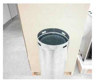
At this stage of the installation the unit is installed with the flue system and any optional kits. The next step is to install and set the nailing strips in the correct position to accommodate the front wall framing and finishing.
