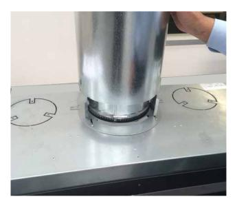
6. The final length of 9" / 11" galvanized flue pipe has ventilation slots at the top where it meets the cowl - to allow heat to escape.
