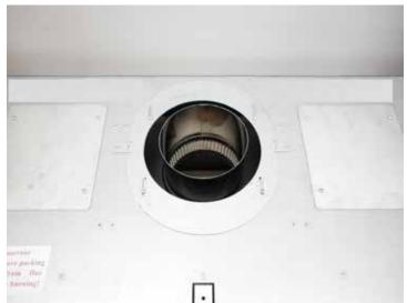
2. Insert the 7" stainless steel active flue. Note: crimped end is down. Must connect active pipe using stainless steel rivets or self drilling screws. 2 for each join.
