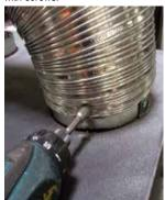
11) Final step is to double check the fan ducting connections at both the unit and fan. Next ensure there is a minimum of <u>25mm clearance to combustibles</u>. Strap and secure the fan duct. Double check the operation of the fan and all electrical work is completed.
