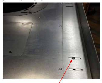
Nailing strip installed with slotted side on unit. The slot allows the movement of the nailing strip to be adjusted depending upon thickness of finish material.
