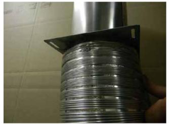
5. Cut a hole on your pre-determined outside wall to allow the fresh outside air hood to be installed. Install and secure the outside air hood. Seal around the flange to ensure tight seal against exterior of home. Join the 150 mm diameter flex duct from the unit adapter to the fresh air hood on the inside of the wall.
