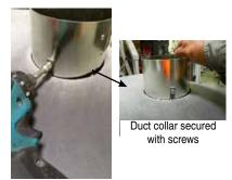
**10)** The fan duct is now ready to be attached to the unit. Slide the ducting over the collar and secure with screws.
