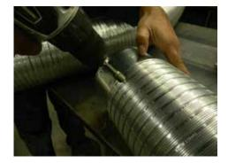
2. Attach the 4.5m duct within this kit to the connecting collar on the opposite end with the screws provided. Extend the flex to the desired length.
