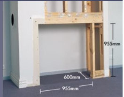
Zero Clearance Box positioned in framework on 12mm sheet
